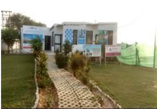
Site Sales Office
