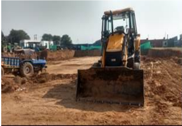
Tower B Excavation in progress
