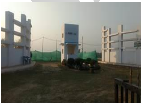
Security Main Gate
