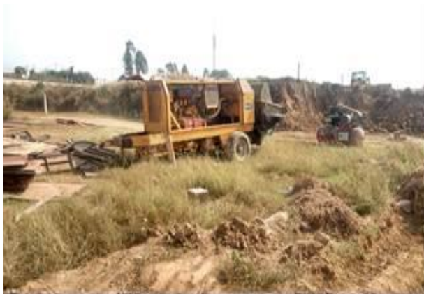
Machineries on site
