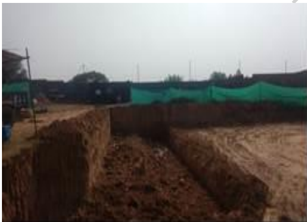
Tower B Excavation and Contractor's site office
